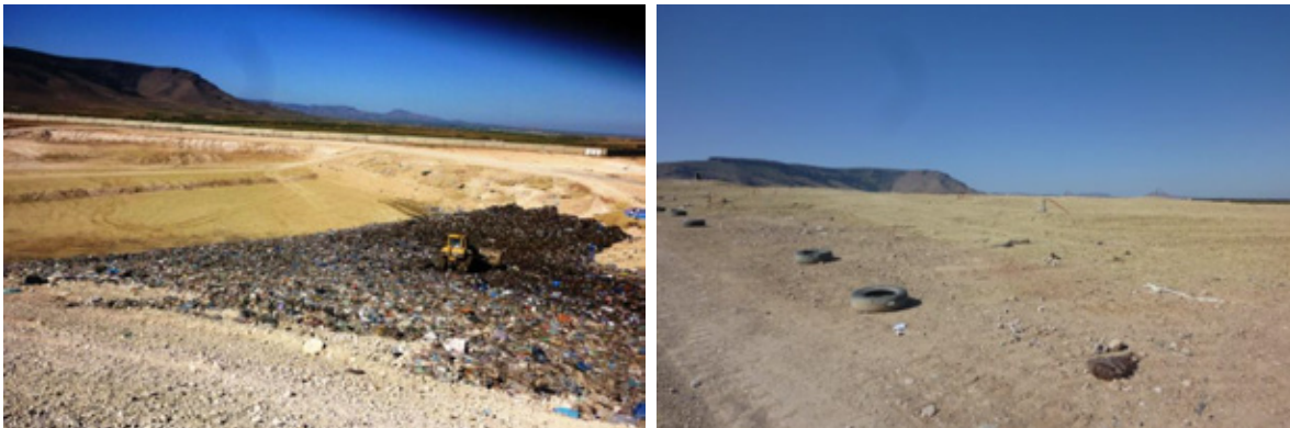
Fresh industrial and domestic wastes being compacted (left) and site ready for vetiver planting
