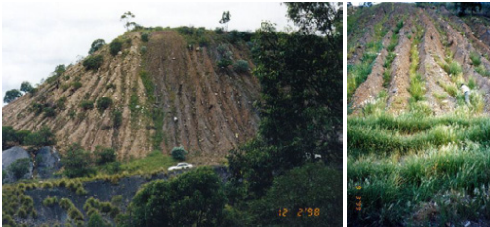
Coal mine waste before and after vetiver planting
