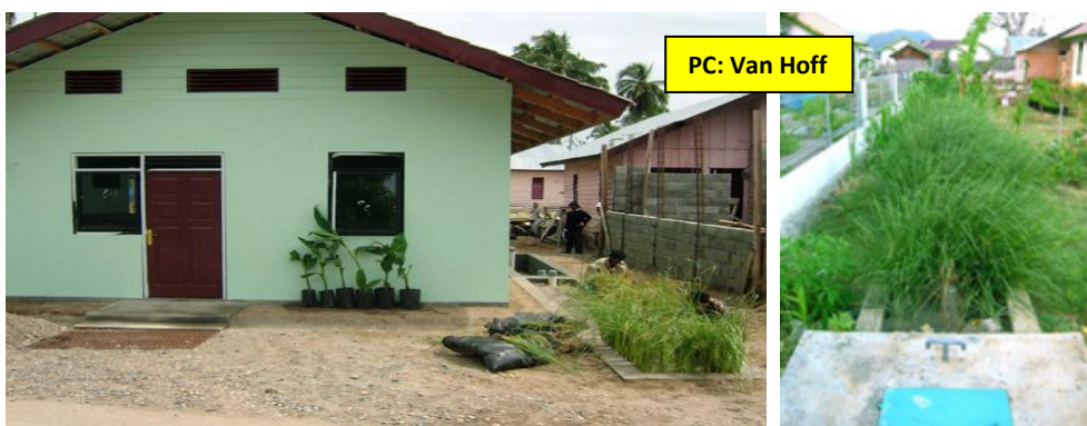
Domestic effluent disposal system using VST in Aceh, Indonesia
